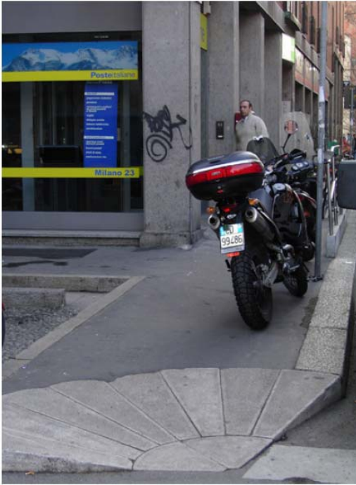
Picture 1. Sloped curb not suitable for blind people and partly obstructed.
